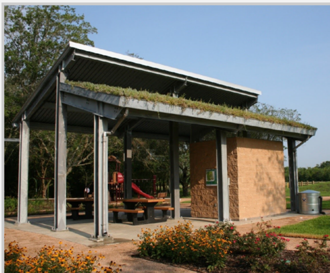
GREEN ROOF ON A PARK PAVILION IN LEAGUE CITY, TX. PHOTO COURTESY OF GIFT - TEXAS A&M AGRILIFE EXTENSION
