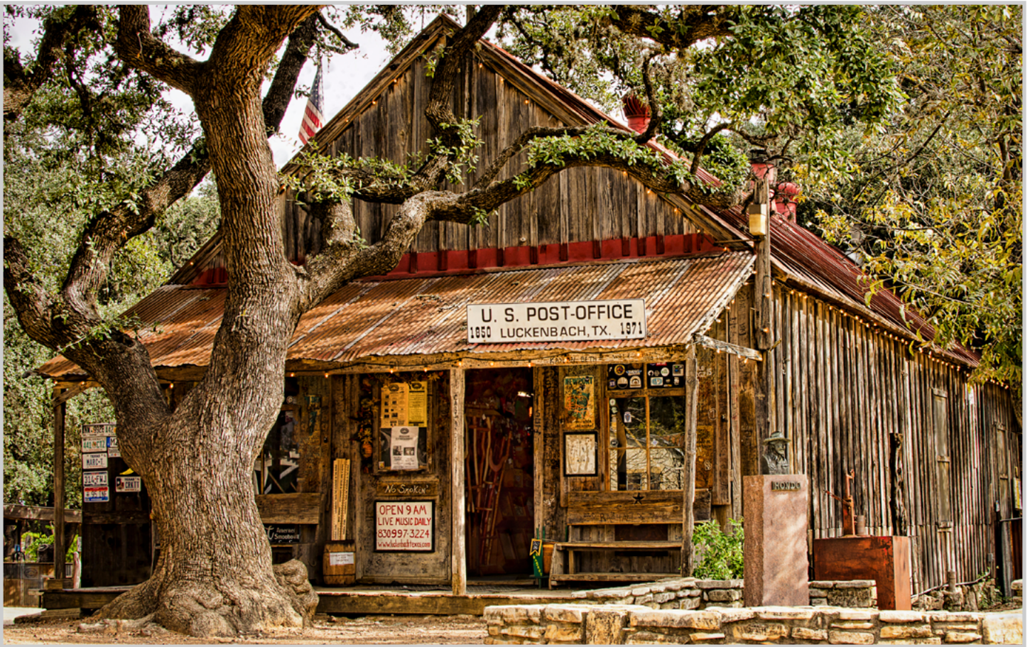
THE HISTORIC LUCKENBACH POST OFFICE OPENED IN 1849. PHOTO COURTESY OF NANCY NAYLOR
