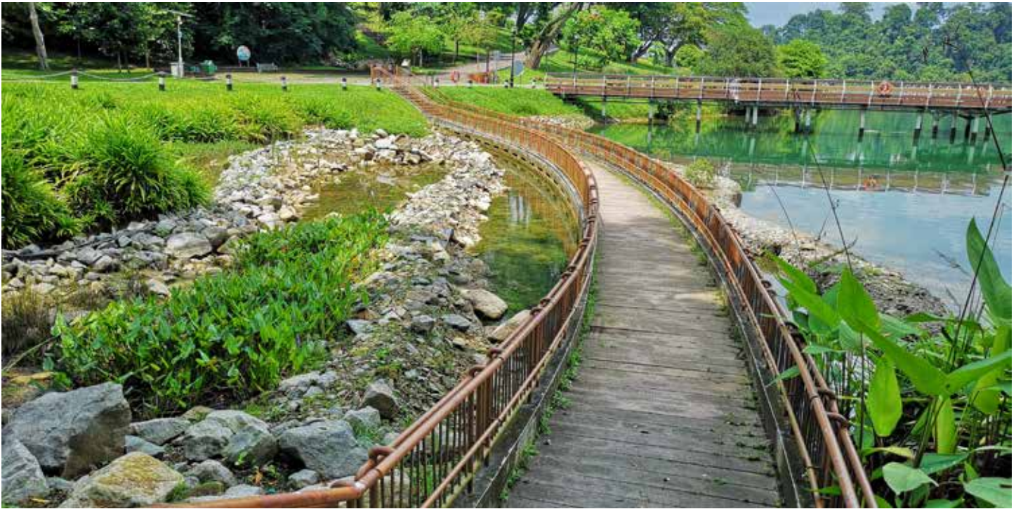
SA bioswale in Singapore's MacRitchie Reservoir Park helps remove stormwater pollutants while adding beautiful green space to a highly urban city.
