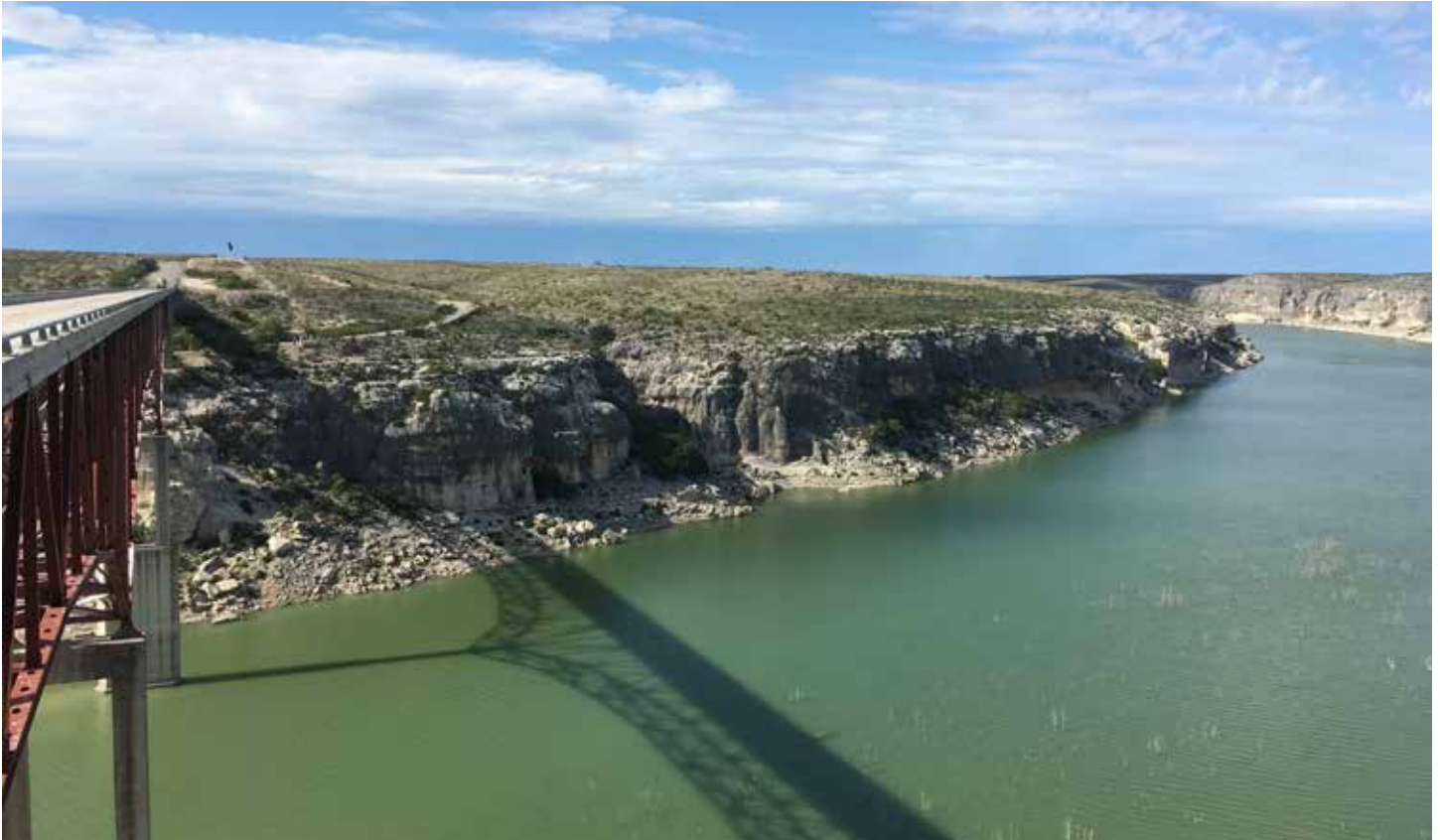
US-90 as it crosses the Pecos River Bridge outside of Del Rio, Texas.
