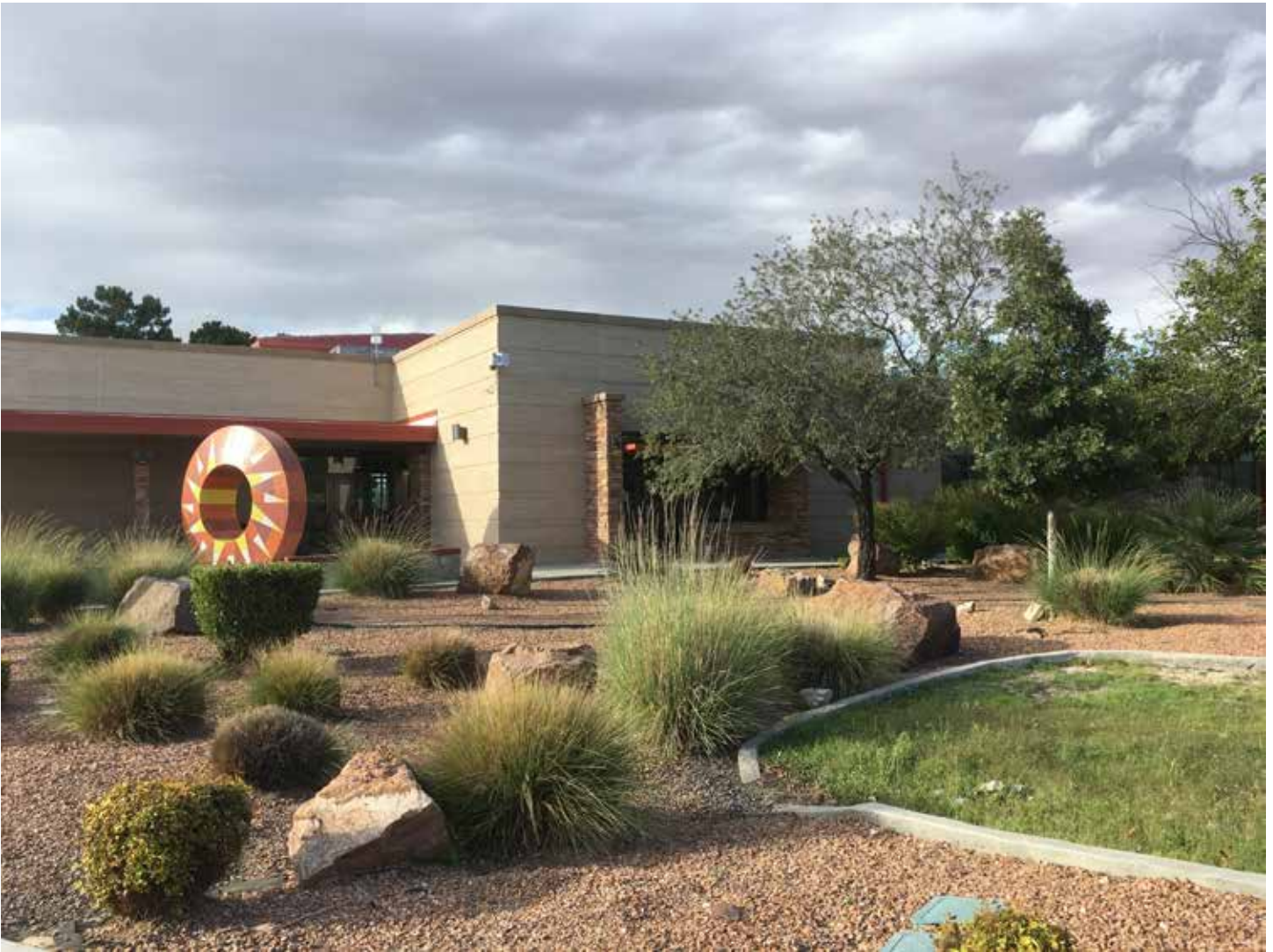
Rain garden outside El Paso Public Library's José Cisneros Cielo Vista Branch.
