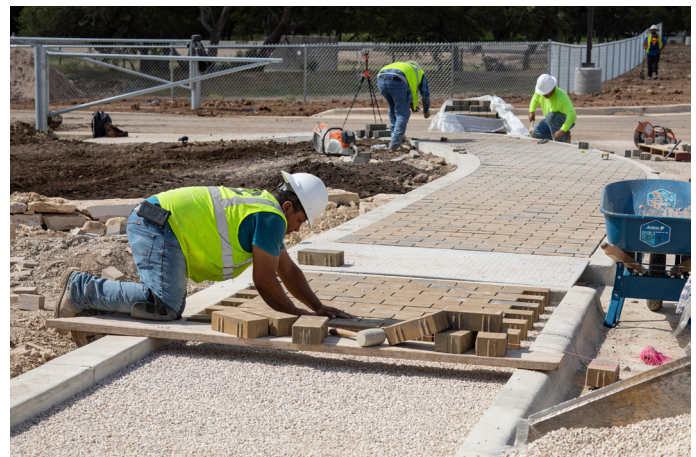
Figure 11: Permeable paver system being installed. Photo by Ray Don Tilley.
