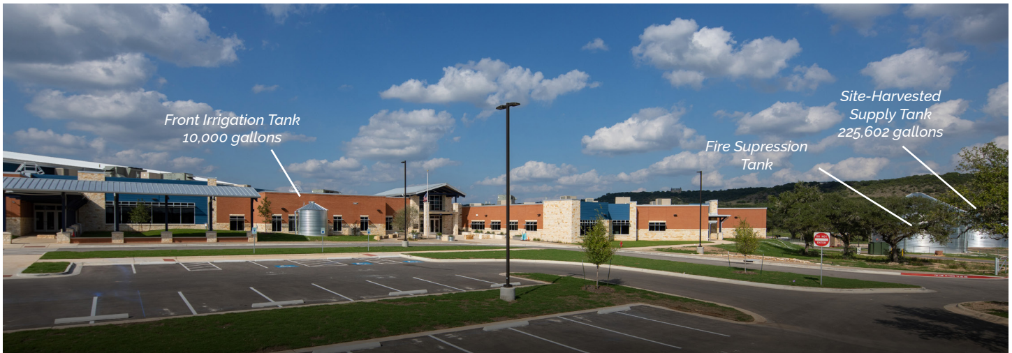
Figure 6: Blue Hole Primary water supply tanks. Photo credit: Ray Don Tilley.
